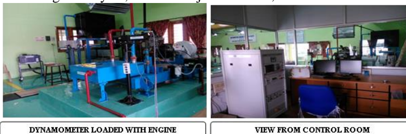
Figure.2. Eddy Current Dynamometer Facility and the E-DAC System
