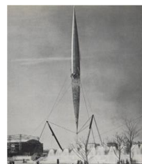
Figure.2. Fuller's mast as a tensegrity structure
