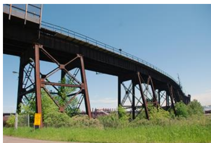
Figure.4. Photograph Of A Plate Grider Bridge
