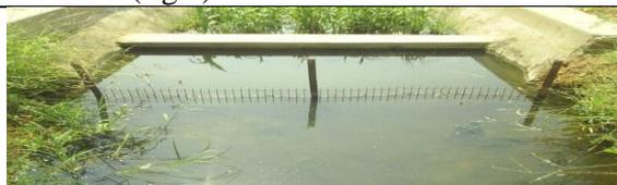
Fig. 1. Inlet zone of the reed bed system
