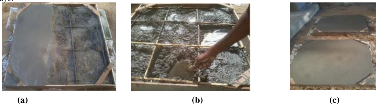
Figure 3a & 3b Steel and bamboo reinforcement
