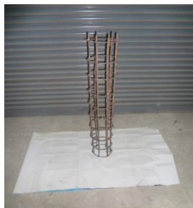
Figure.1. Column reinforcement
