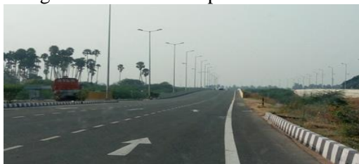
Figure.6. Safety Sign and Service Road
