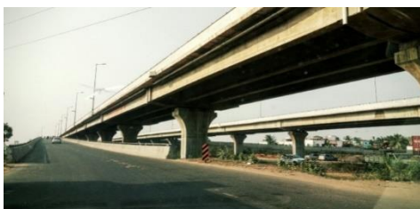
Figure.3. Nemilicherry, ROB Flyover, outer ring road, Chennai
